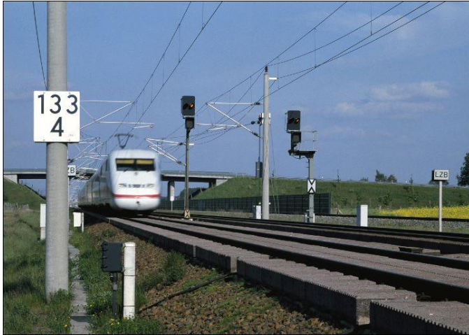
Figure 10: High- speed railway track Hannover - Berlin (Source: Bahn im bild)
